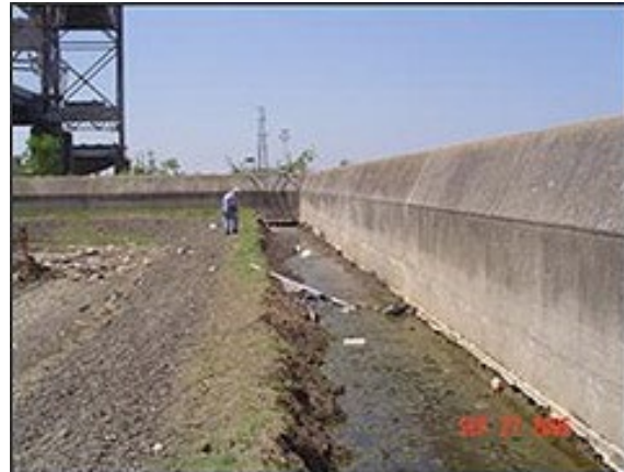
Figure 9. Effects of Scour Near the IHNC
